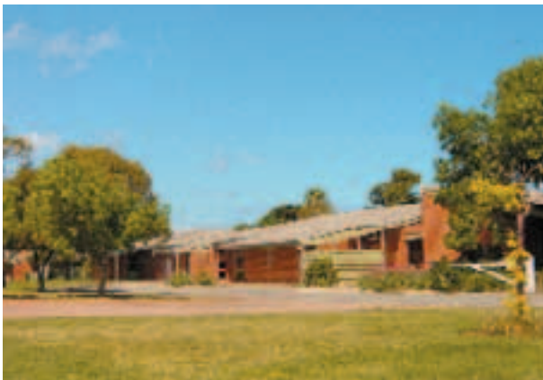
The now vacant site of the former Townsend School
